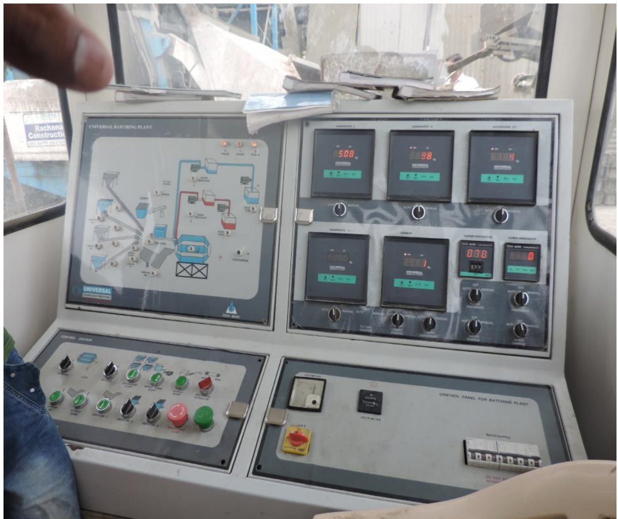
Control Panel for Batching Plant at Sachin
