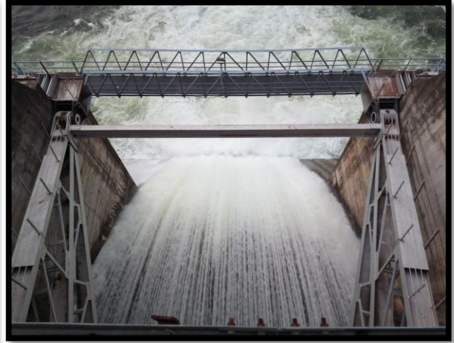
Spillway of Dam
