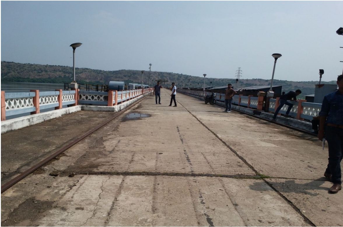
Kadana Dam site
