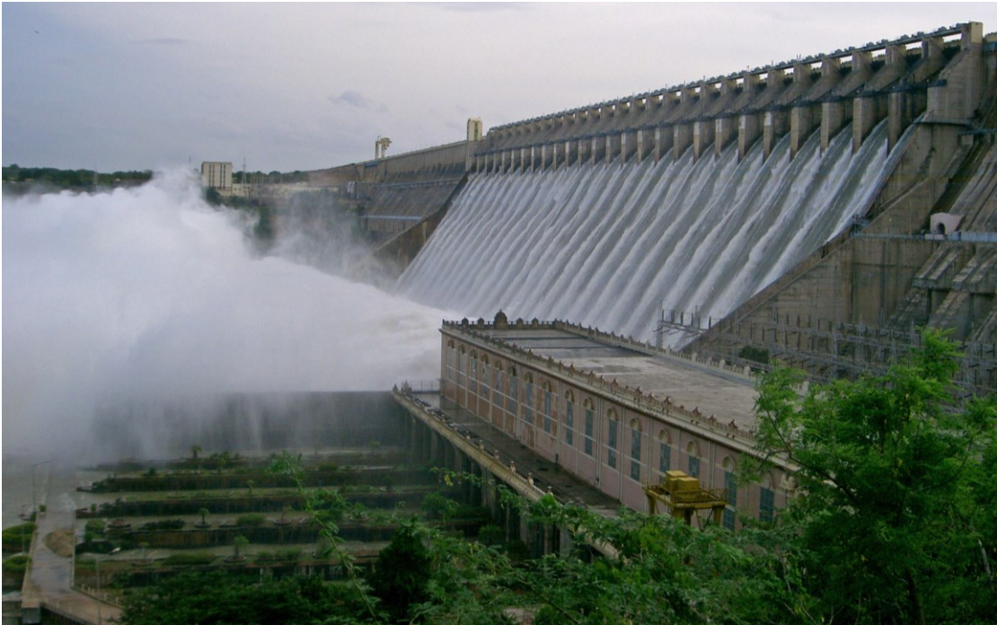
Water flowing through Gates'
