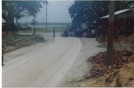
Fig. 4. JGT laid on subgrade
