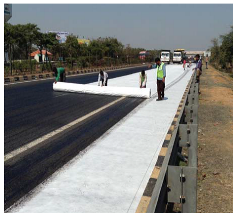
Fig. 6. Installation of paving fabric (courtesy: TechFab India Industries Ltd.)
