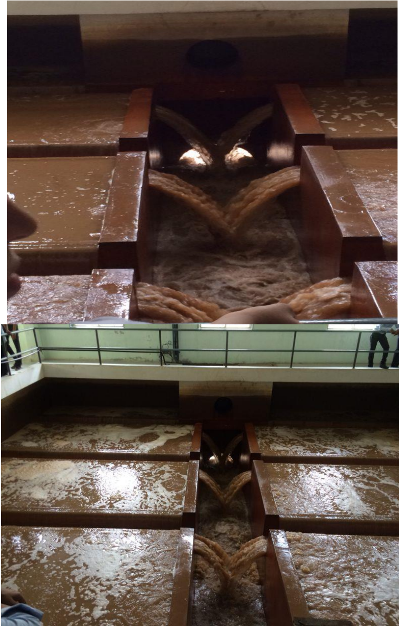
Backwashing of sand filter
