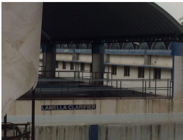
Lamella Sedimentation unit
