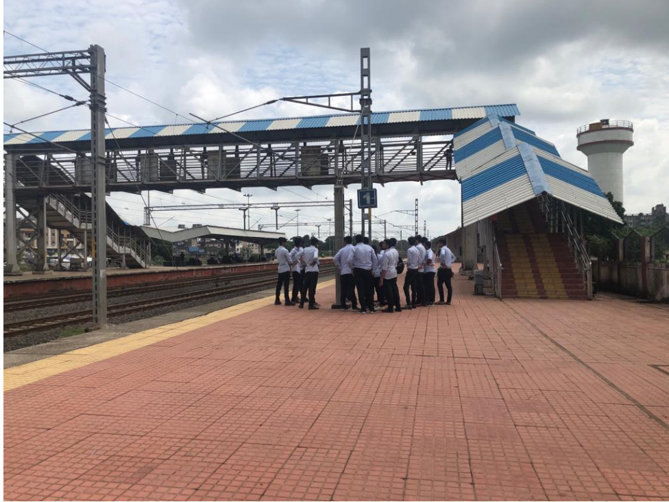
Steel foot over bridge
