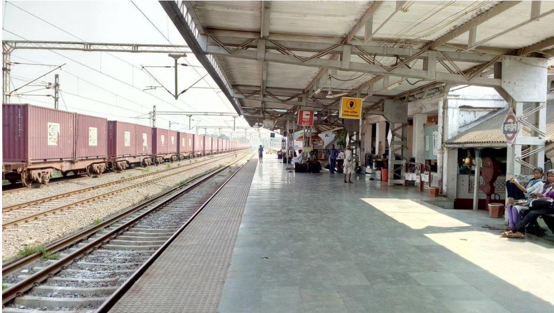
Cantilever roof at Railway Platform of Bardoli Station
