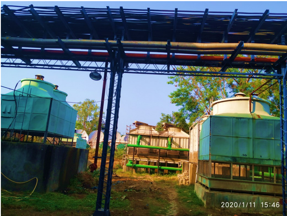
Solar operated vapour absorption chiller
