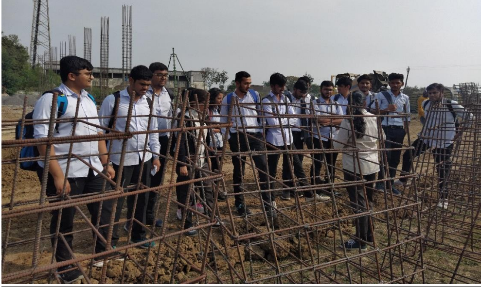
Student observed reinforcement cage of pedestal
