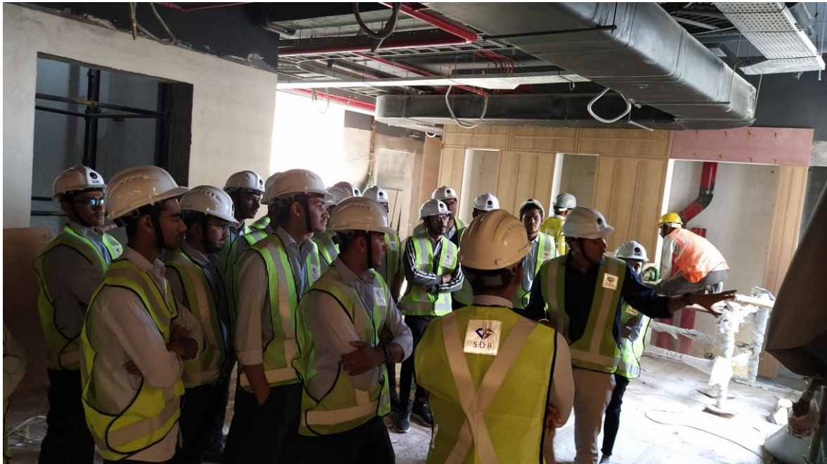
Explain about different building services which installed in SDB
