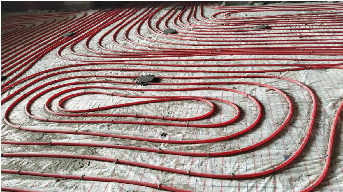
Radiant cooling system which is installed in central spine corridor
