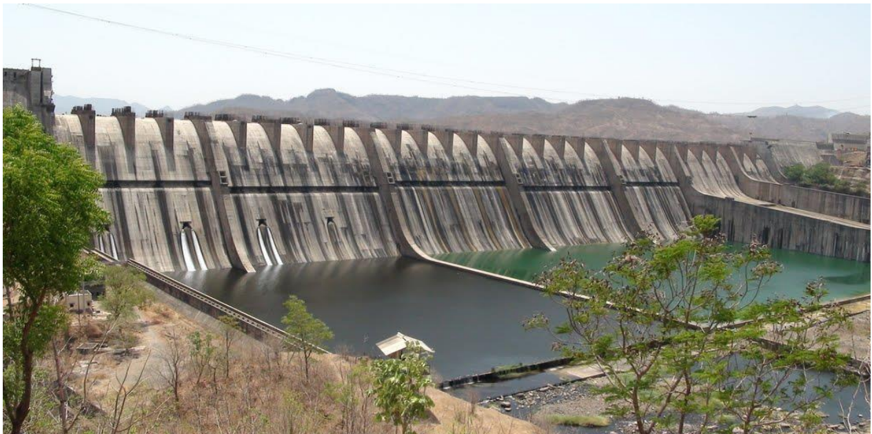
Hydro power plant
